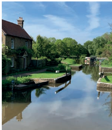
Walsham Gates with the river beyond and Walsham Weir round to the left of the cottage
